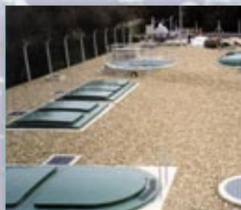
Individual primary, biological and secondary treatment units which can be used to construct very large treatment works.
