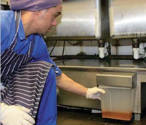
Fatstrippa is fully compliant with both the letter AND the spirit of The Building Regulations (part H 2.21) which state, "Drainage serving kitchens in commercial hot food premises should be fitted with a grease separator...effective means of grease removal."
